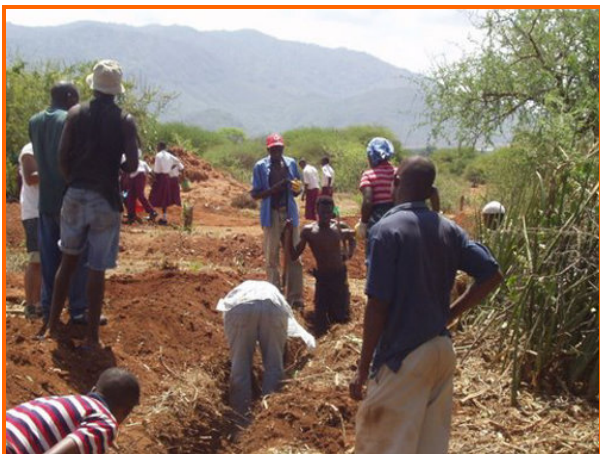
Foundations for schoolroom, Mwanga, Northern Tanzania, November 2007
